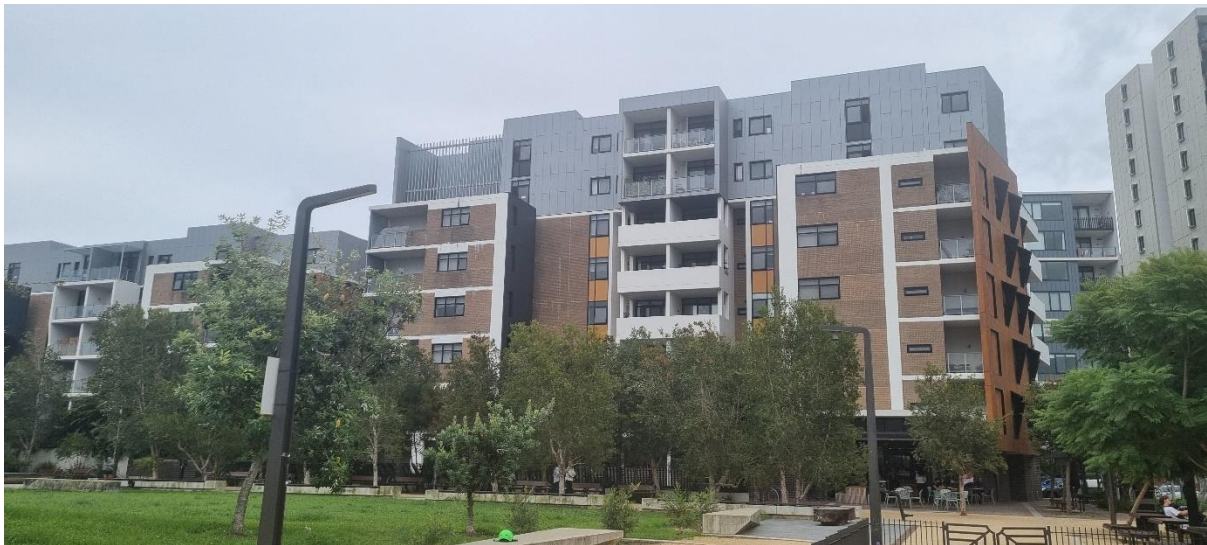
Figure 7: Adjoining residential flat buildings towards the southwest of 'Banga Shed'
