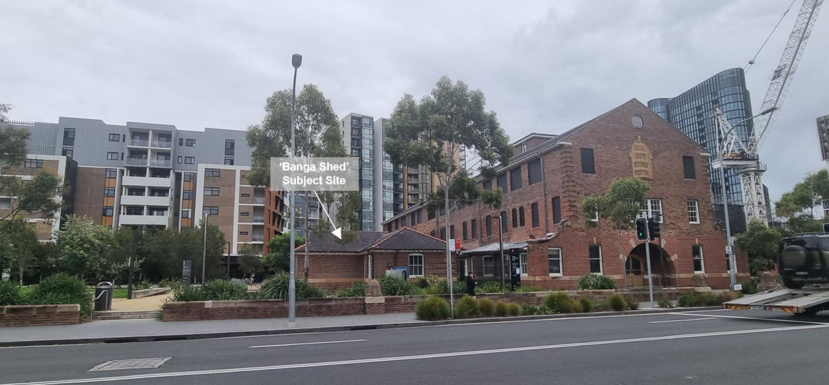
Figure 2: Site viewed from Joynton Avenue facing west
