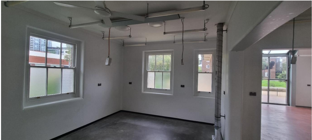
Figure 4: Eastern internal space within 'Banga Shed'
